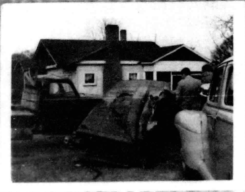
Right side of Horizontal stabiliser
